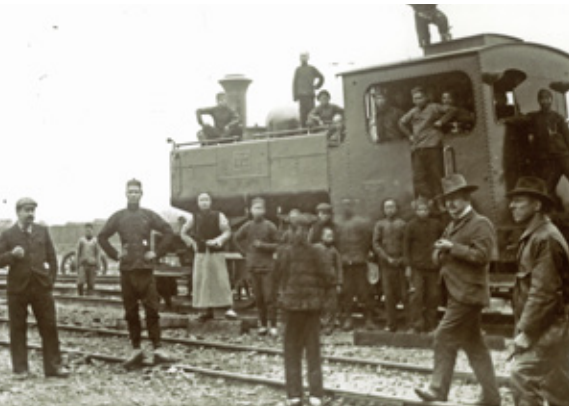
Construction of the Beijing-Hankow railway, China (ca. 1903).
