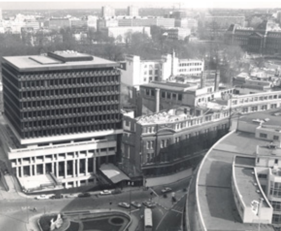
The reconstruction of the headquarters on Rue Montagne du Parc occurs in two phases between 1966 and 1978.
